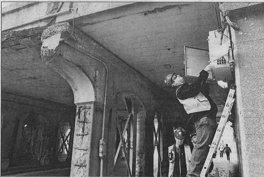
Research Engineer Mat Kotowsky finishes work on a wireless transmitter, which is part of a system of stress sensors on the CTA viaduct over Sheridan Road near Devon Avenue. CHRIS WALKER/TRIBUNE PHOTO
