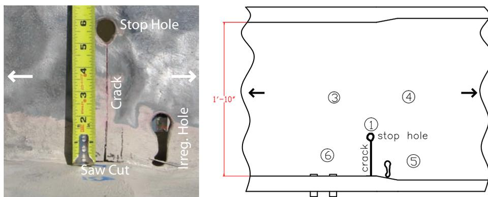
**FIGURE 1.** Annotated photograph (looking down) and drawing of flaws on horizontal web of top chord: 5” long transverse crack, stop hole, partial-depth saw cut, and irregularly-shaped hole. Circled numbers represent transducer locations. Heavy arrows indicate axial tension in the member.
