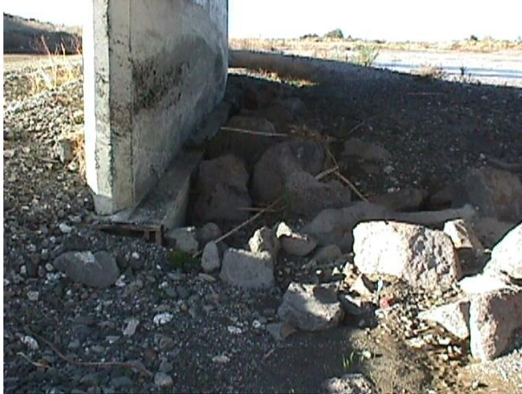
**Figure 1:** Scour pocket along, rather than at the upstream or downstream end of, a bridge pier
