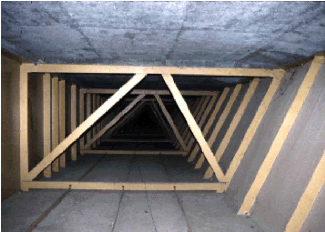
Figure 1. Typical Crossframe.
