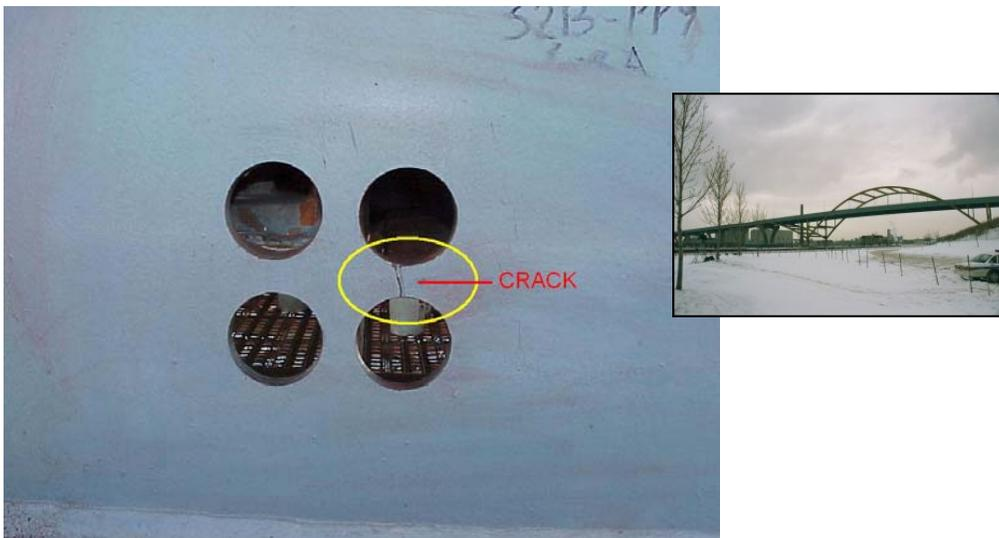
Figure 1: A bridge with a crack
