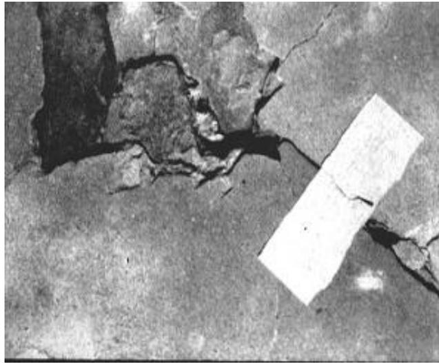
**Figure 1: Crack in Mortar Coat Over Rubble Stone.**
