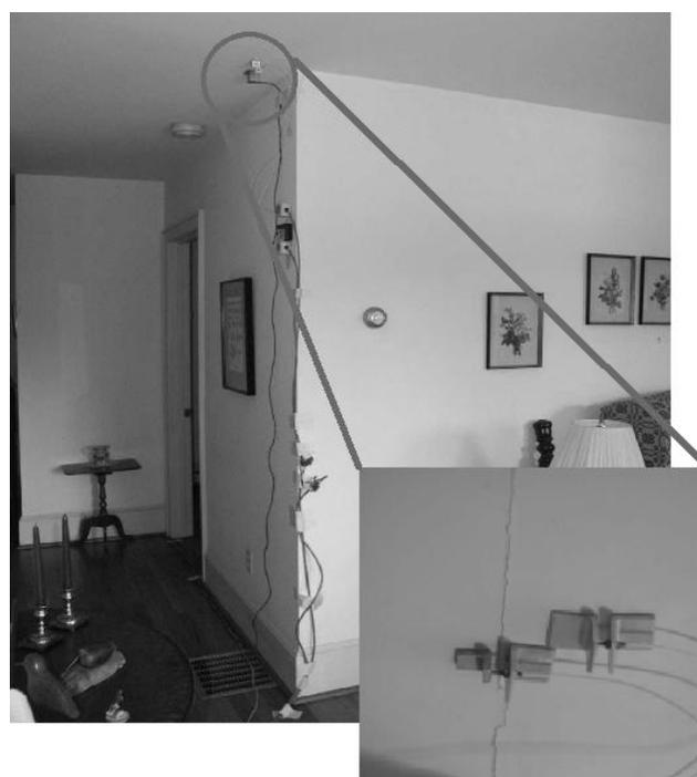
Figure 3. Photos of sensor and crack 1
