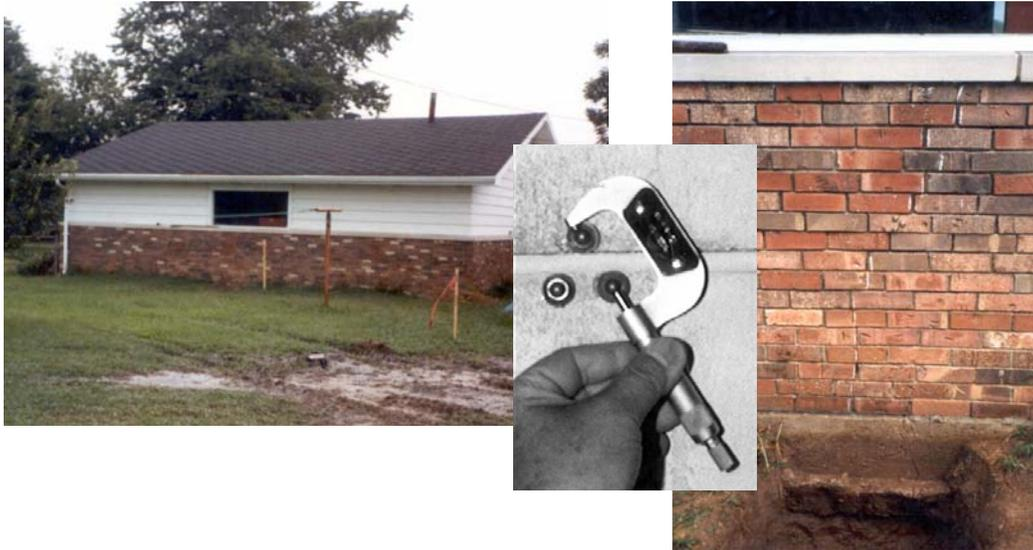
Figure 8 Slab-on-grade garage (left), outside crack (chalk line on right photo), and micrometer and measurement points to sense shearing as well as opening and closing.
