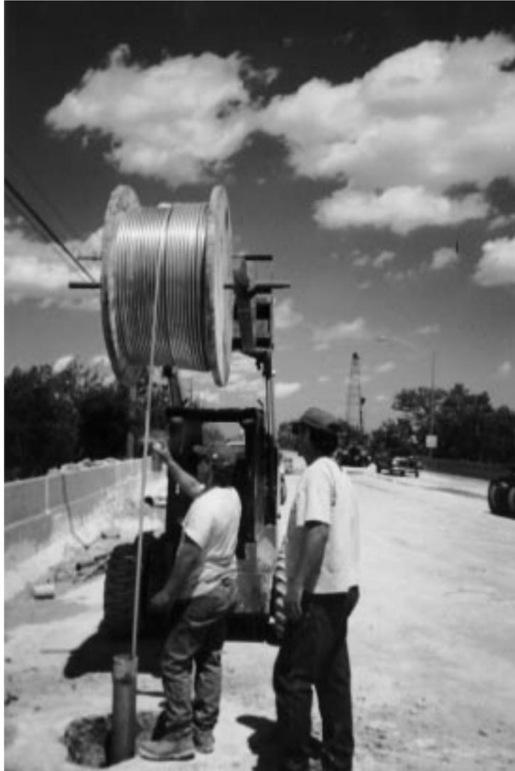
*Figure 10. Installing coaxial cable in a rock pedestal supporting a highway.*
