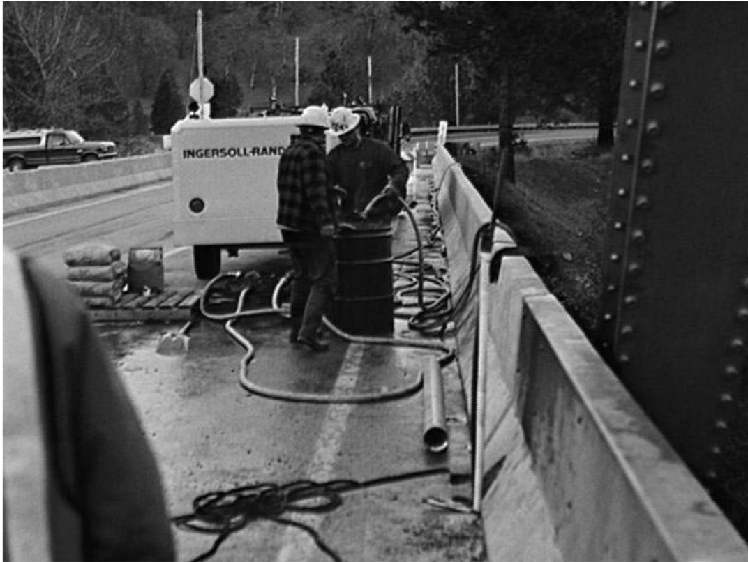
Figure 8. Installing cable from bridge deck. Preparing to pump grout through PVC tremie pipe.
