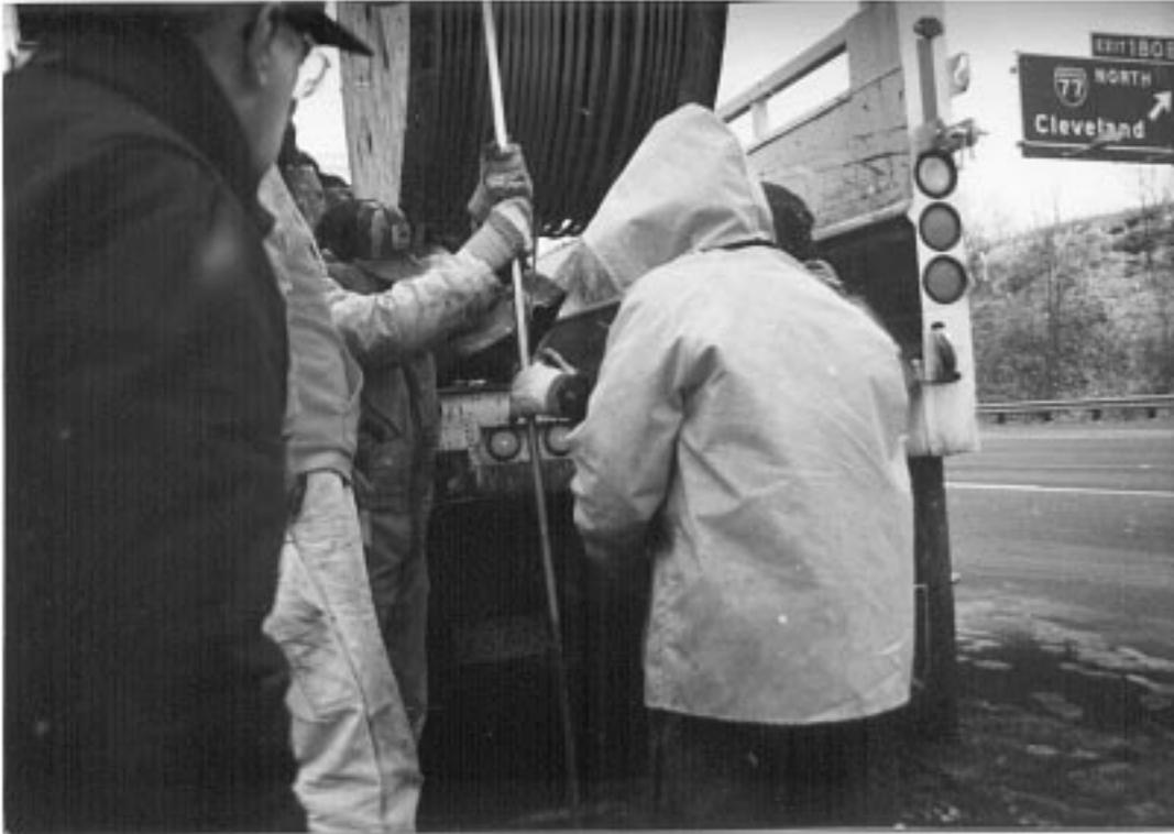
*Figure 5. Installing coaxial cable in hole drilled into an abandoned mine in Ohio.*
