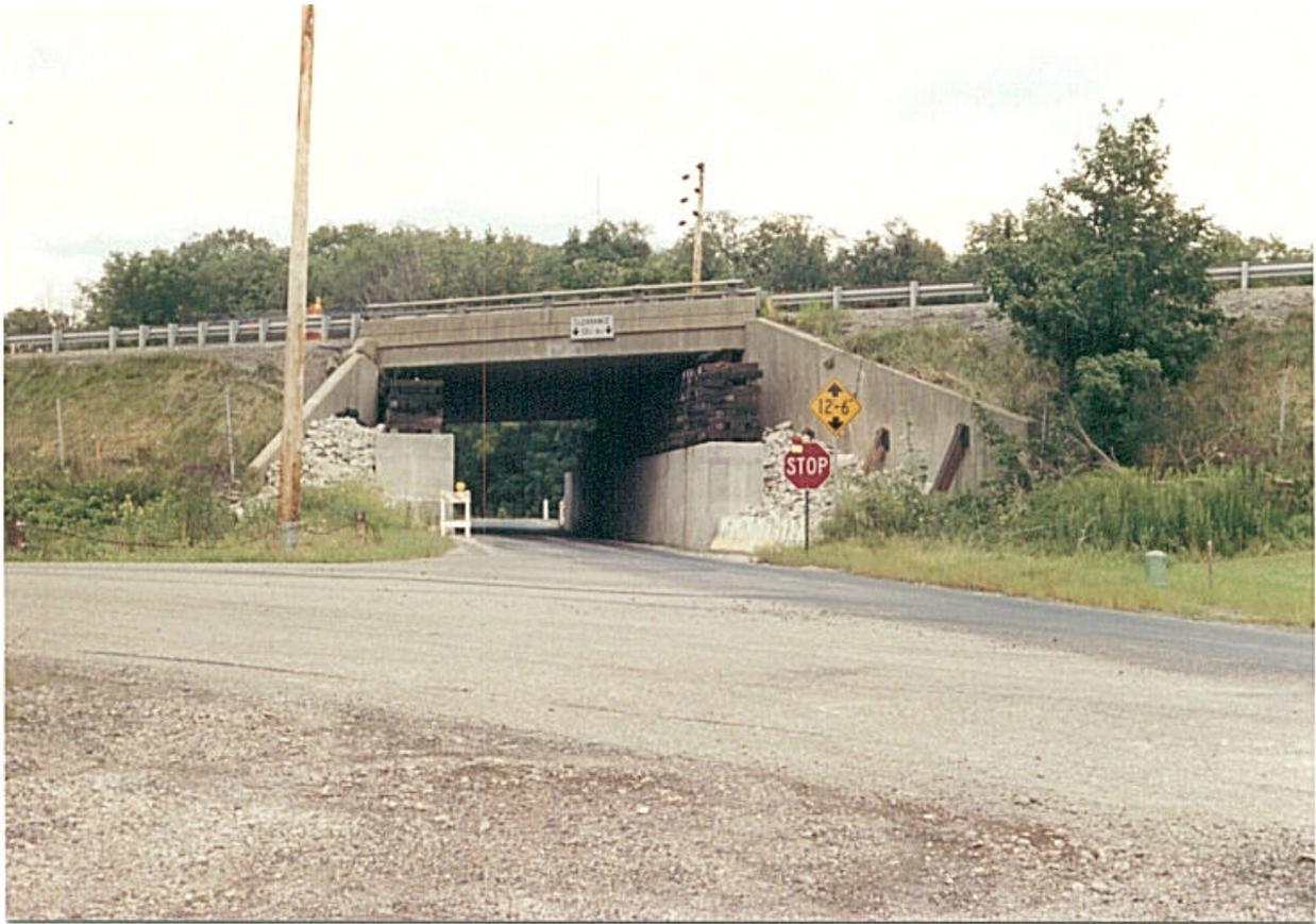
**Figure 2. View looking northeast at Zedeker Road overpass. The cast-in-place reinforced concrete blocks and wood cribbing were placed to provide additional support for the bridge deck. TDR-7 is located at the enclosure on the right side of the road.**
