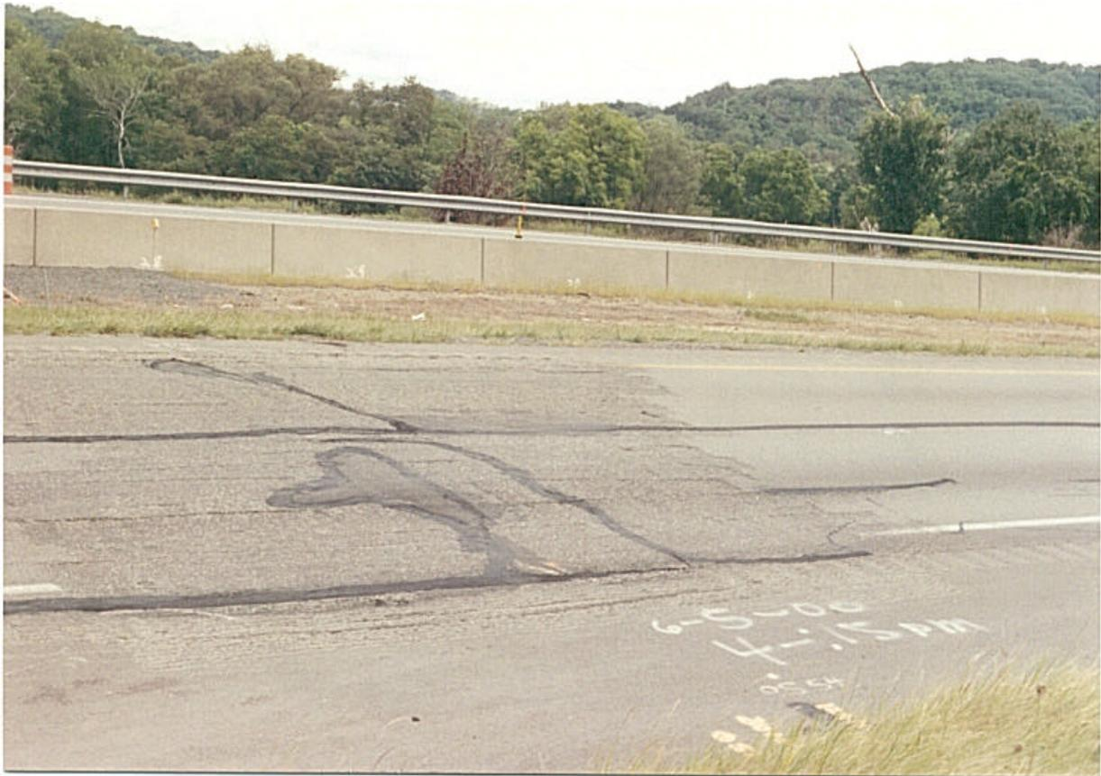
**Figure 10. View looking northwest at the location where the 12 mm high compression bump developed. The asphalt was ground down to relevel the road surface.**
