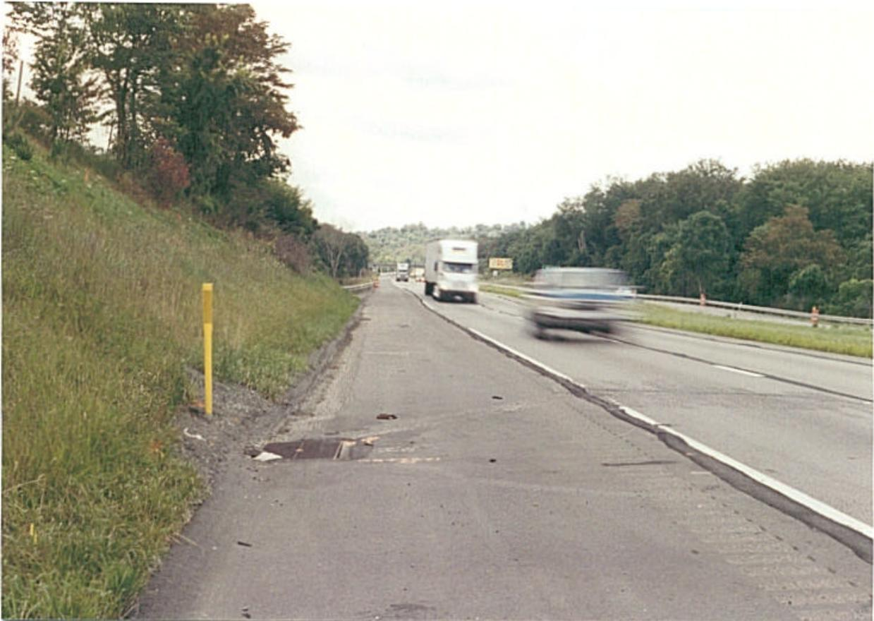
**Figure 9. Margin of final subsidence trough over the south edge of Panel 4 South. Note the guardrail in the right of the picture.**
