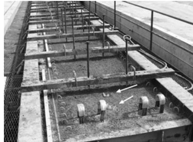
Fig. 12. Field measurements on box girder shortly after placing the concrete
