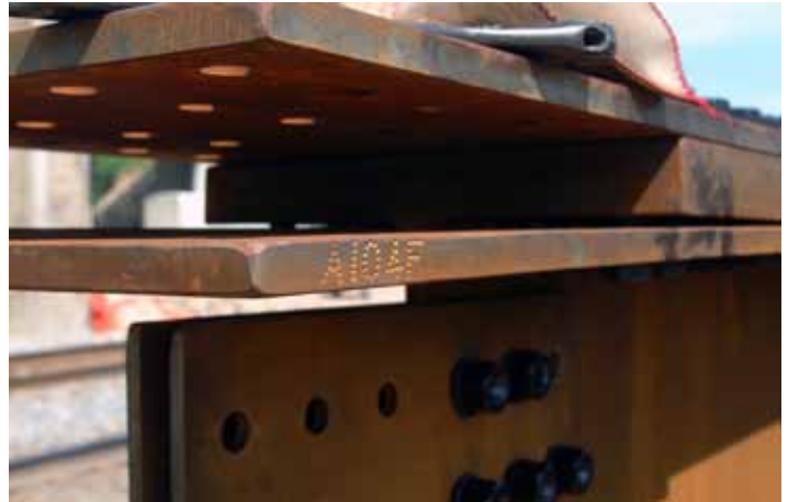
ITI-developed A710 Grade B steel bridge components awaiting installation
