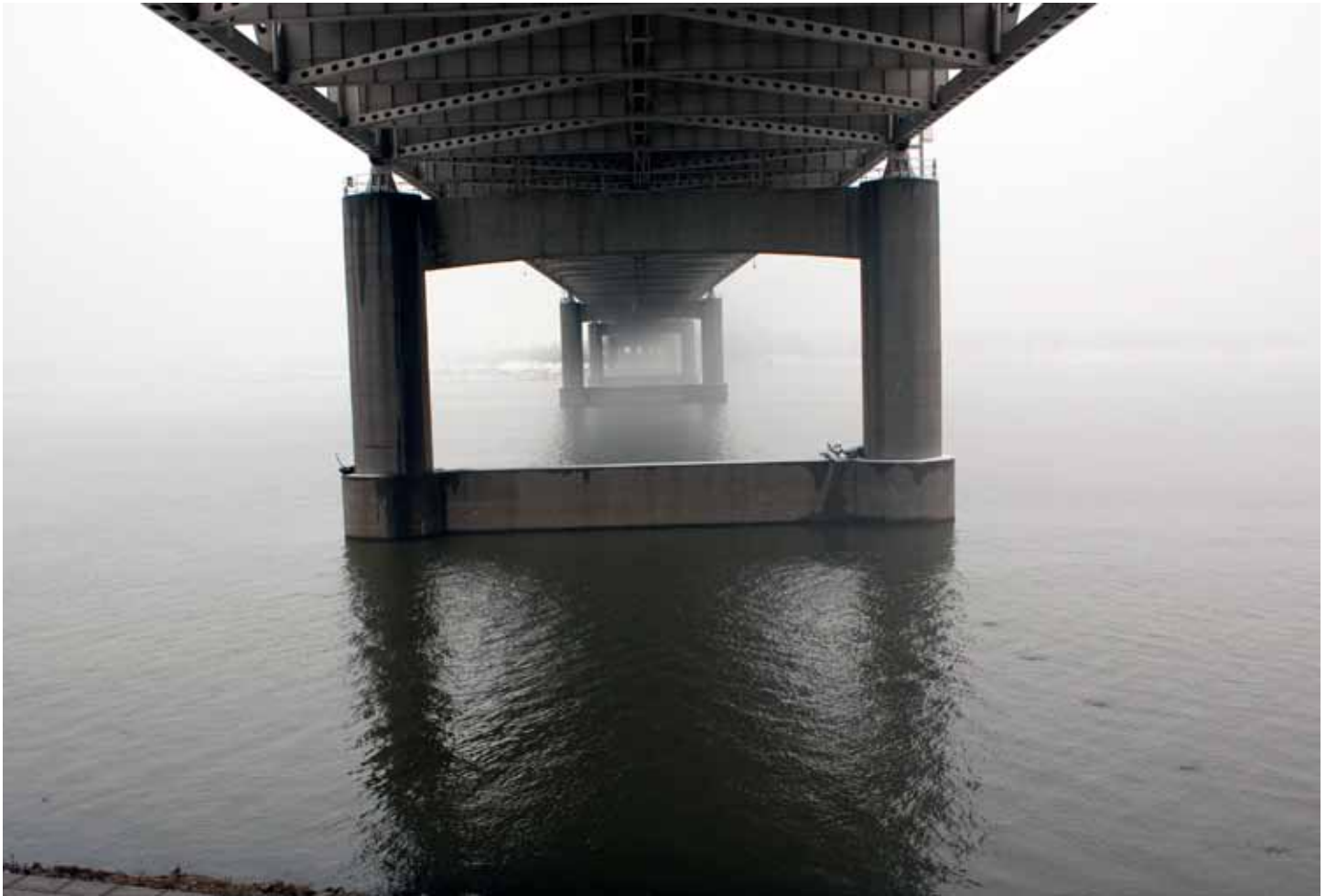
The John F. Kennedy Memorial Bridge carries Interstate 65 over the Ohio River at Louisville, Kentucky.
