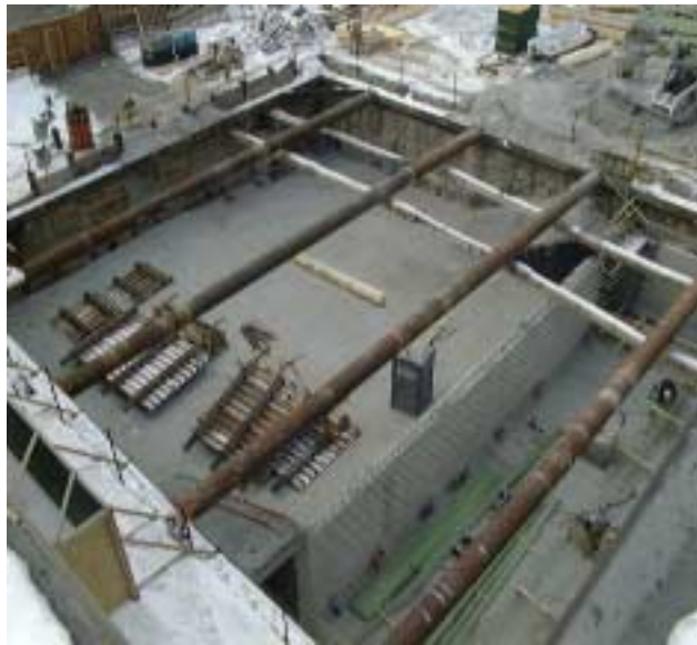
Figure 1. Excavation to First Tieback Level
