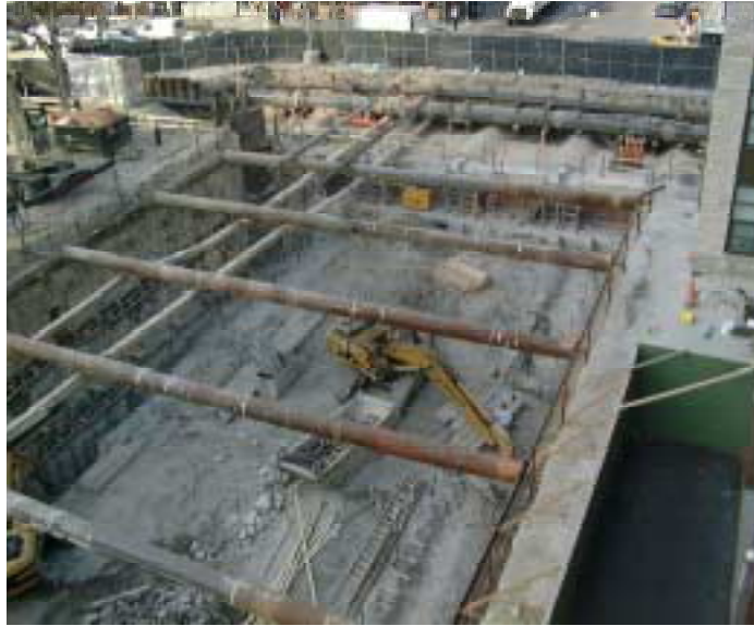
Figure 1. Excavation to First Tieback Level
