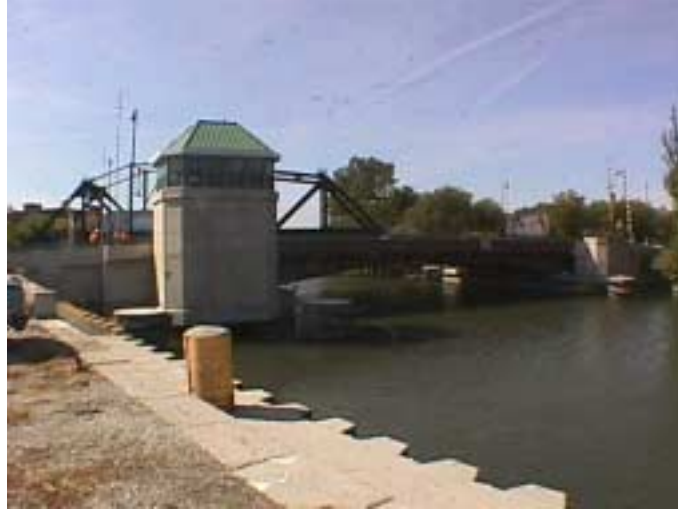
Figure 17. Kinnickinnic Lift Bridge, Milwaukee, Wisconsin
