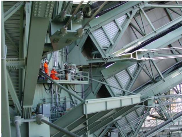
**Institute engineers installing AE sensors on thrust bearings in Miller Park, Milwaukee, Wisconsin**
