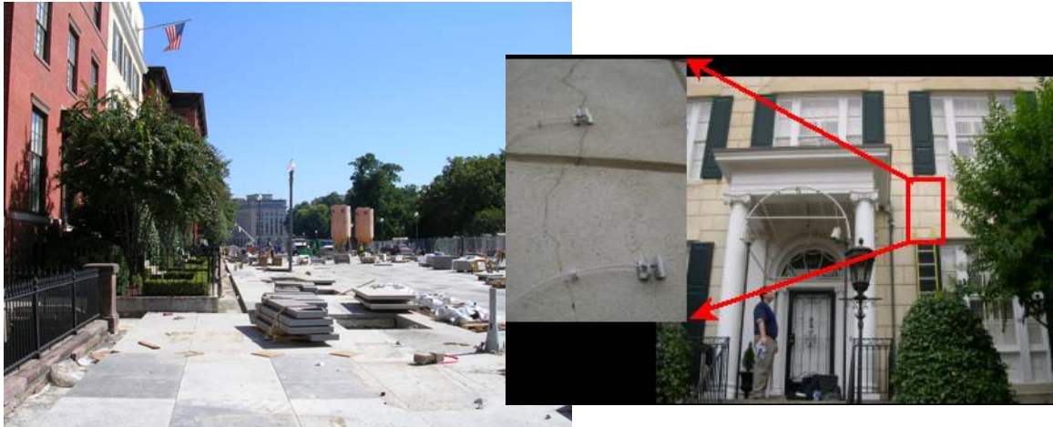
Blair House TDR installation
