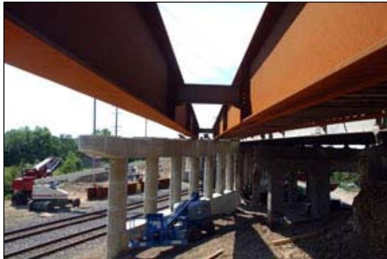
Figure 4. Photographs taken during fastening of the steel girders to the concrete supports of the bridge
