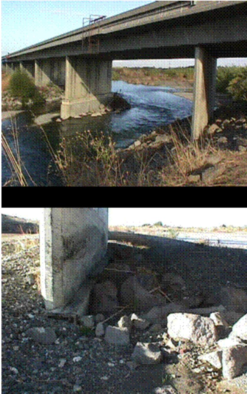
**Figure 7:** Bridge scour at the Stony Creek Bridge. Top: Stony Creek flowing past one of the concrete piers. Bottom: A scour pocket partially refilled with debris. The piling has been partially exposed, dangerously destabilizing the pier.
