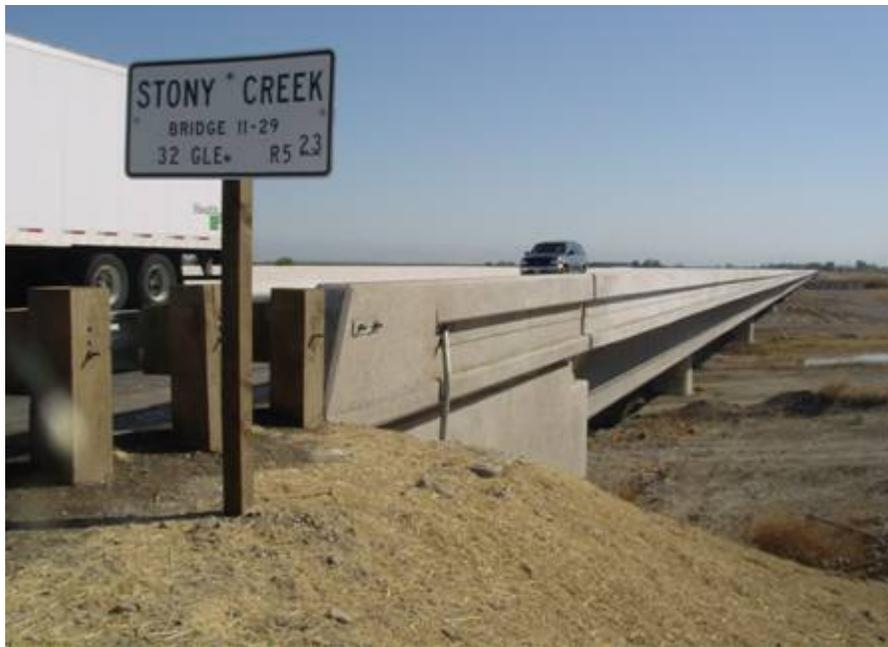
**Figure 6:** Stony Creek Bridge. The bridge passes over a wide creek bed, supported by 19 piers. The location, direction, and strength of the Stony Creek are variable and erratic within this creek bed.
