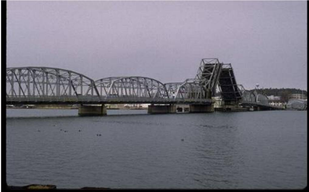
**Figure 1:** The Michigan Street bridge, with the bascule spans in the upright position to allow a ship to pass through the Sturgeon Bay Ship Canal.
